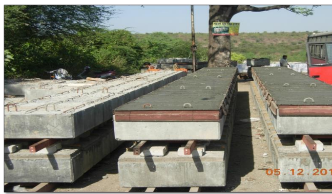
Fig. 1: Manufacturing of wedge shaped blocks concrete strips in the workshop near to site
