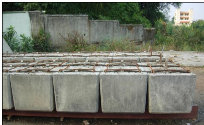
Fig. 1: Manufacturing of wedge shaped blocks concrete strips in the workshop near to site
