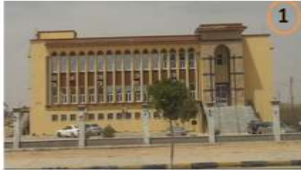
Housing, utilities and environment building
