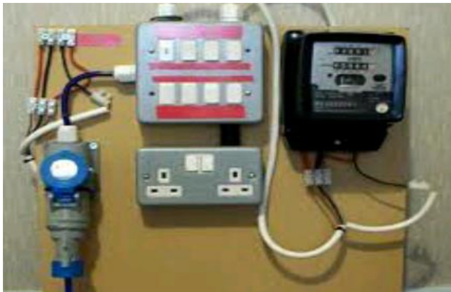
Fig.5. Fitted Prepaid Electricity Meter in Domestic Homes
